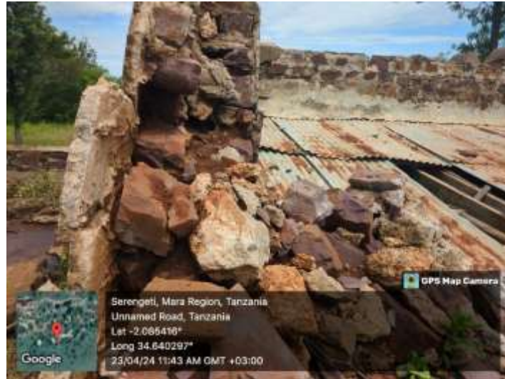
Figure 6: A collapsed superstructure stone masonry wall.
